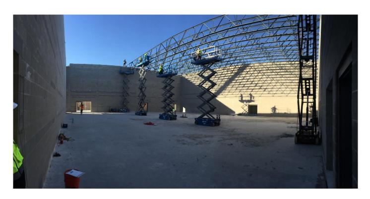
**STRUCTURAL** – Steel roof joists are being lifted and welded into place at the Auxiliary Gym.
