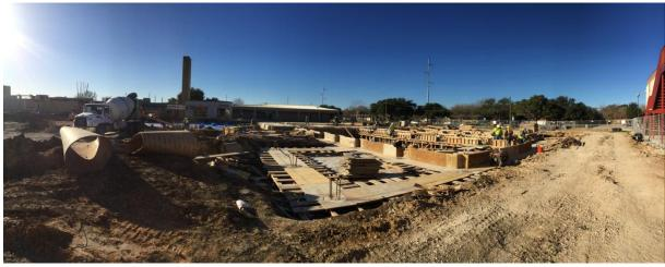
**PIERS/FOUNDATION** – Piers have been drilled and poured at Area E and the form work for the foundation has started. Concrete pours have been scheduled for this area on February 12.
