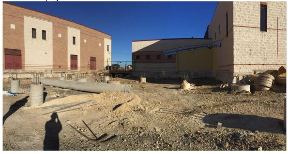
**PIERS** – The pier drilling work has been completed. Steel casing (pipe) was used on 694 of the 813 piers due to groundwater being encountered. The area between the Freshman Center and the Band Hall will house a Classroom, entrance to the ROTC Dept. and Custodial Support Services.
