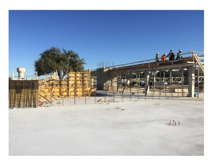
**CONCRETE STRUCTURE** – Formwork is being erected for the concrete beam that will support the 2<sup>nd</sup> level (back wall) of the Performing Arts Center and the upper level seating structural.
