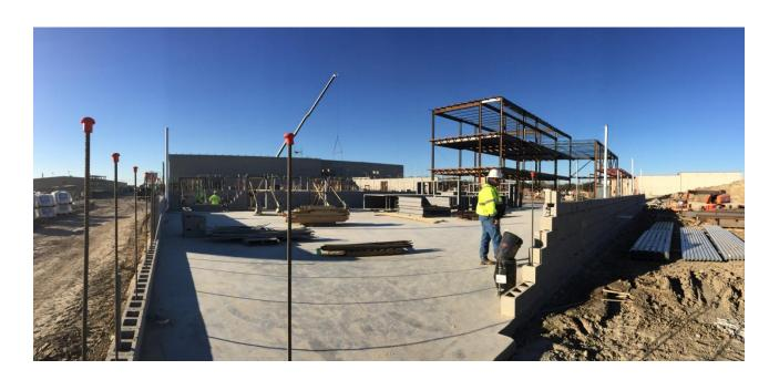
**INTERIOR** – Door frames are being installed prior to block walls being laid. Interior block wall installation is in progress at the new Weight Room, the Trainer's area and the Athletic areas. The structural steel structures on the right will house Classrooms and Large Group Instruction (LGI).
